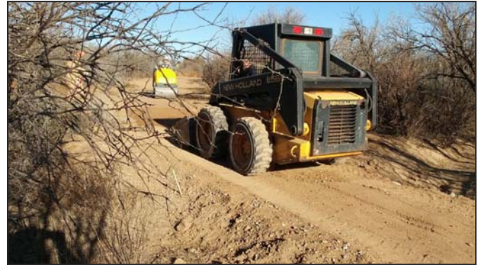
Work on the trail began with leveling and clearing the pathway.
