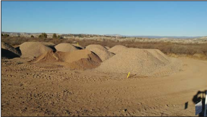
The Yavapai-Apache Nation donated 350 tons of trail base material to the project with an estimated cost of over $5,000.
