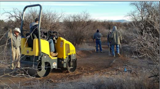
As the trail material is laid down, the volunteers grade and level the materials. A rented roller then compacts the base material.
