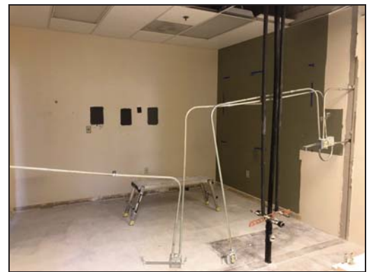
Wall between two examination rooms comes down to create a larger exhibit space.
