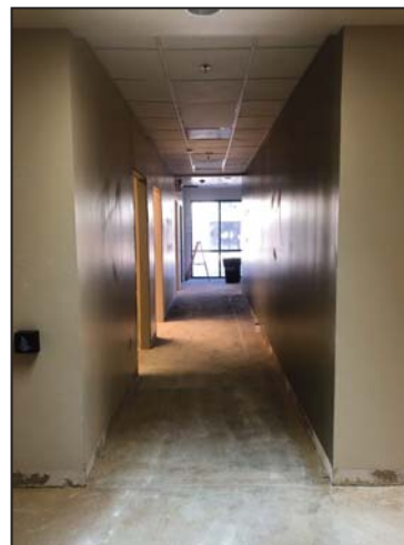
Hallways and rooms are cleared of carpet and tile.
