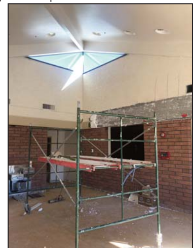
Wall for lobby mural is prepared to provide a smooth surface.
