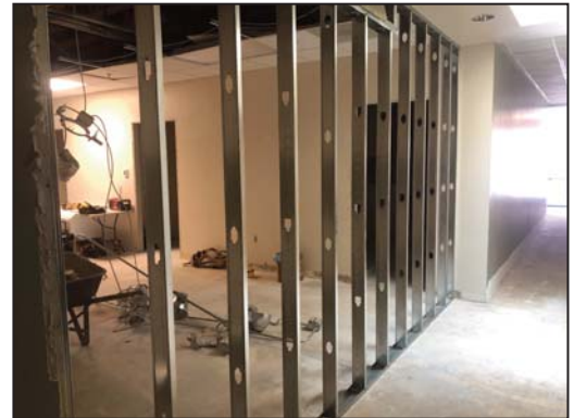
New wall goes up between the museum and administrative areas
